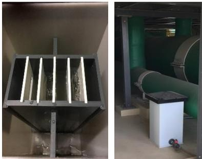
The Ecodosing chlorine dosing regime was implemented in November 2017. The required amount of chlorine dosed could be reduced with 50% in comparison to an effective continuous chlorination. A biofouling monitor was installed to provide operators with real time insight into any risk for biofouling settlement.
