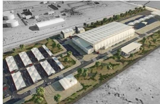
The desalination plant was completed by late 2017. It will supply 60,000m<sup>3</sup> of desalinated seawater a day to the city of Al Khafji in north-eastern Saudi Arabia, providing a regular supply of water to the region throughout the year. The facility will employ the new Solar Saline Water Reverse Osmosis (Solar SWRO) desalination method using ultra-filtration (UF) for the pre-treatment process.
